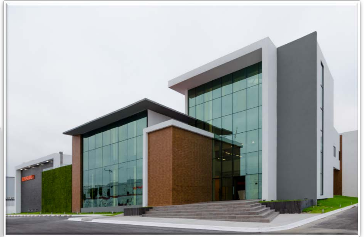
Above: new premises constructed in Apodaca, Mexico.
